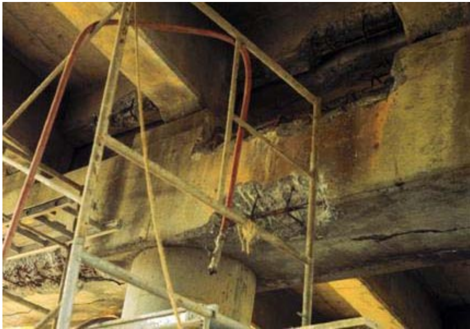
FIGURE 2. Typical Bridge, I-81 Interstate, Virginia – Close-up of Pier Cap Deterioration.
