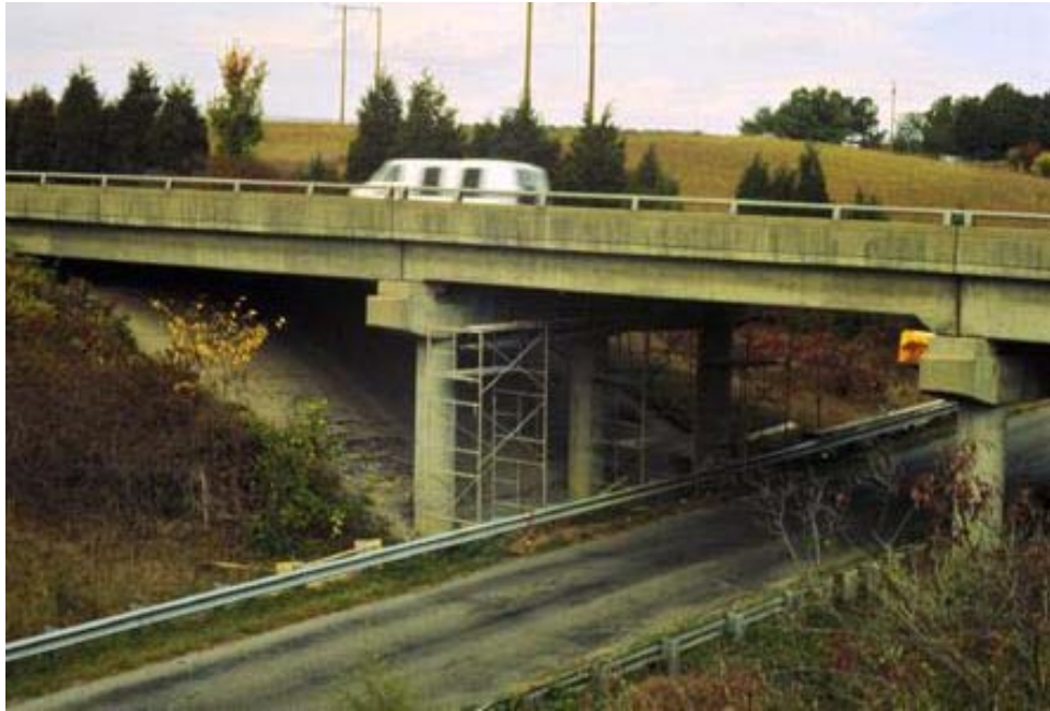
FIGURE 1. Typical Bridge, I-81 Interstate, Virginia – Pier Cap Deterioration
