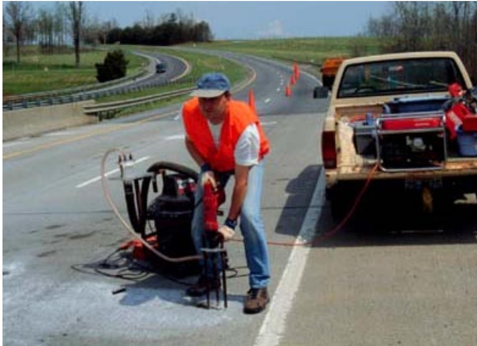
FIGURE 6. Sampling for Chloride Concentrations – Collection Apparatus: Impact Drill with Hollow Drill Bit, Powder Concrete Collection Unit, and Vacuum.
