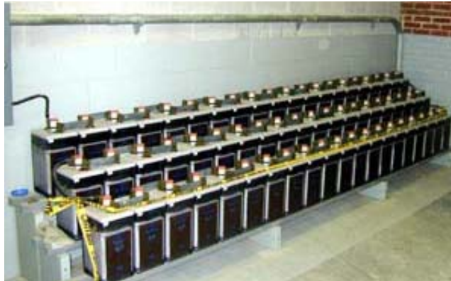
Figure 8 Backup batteries in the substation
