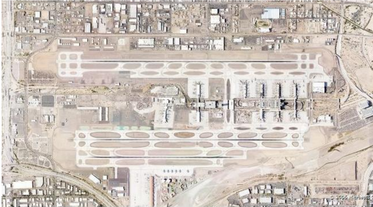
Figure 39: Aerial Photo of Phoenix Sky Harbor International Airport (Photo Courtesy of Microsoft).
