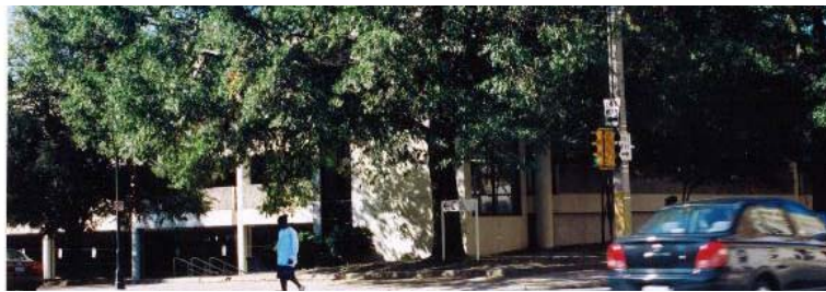
8. 1980, VCU Main Street Parking Deck
