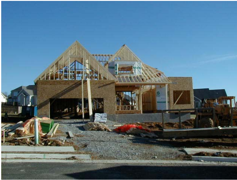
Figure 1.1: Light-frame structure under construction.
