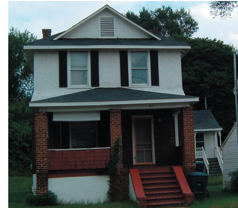
A typical house with porch in the community of the chosen site. (photo is taken by the author)
