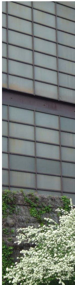
ELECTRICAL SUBSTATION WASHINGTON, DC OWNED BY DOMINION VIRGINIA POWER
