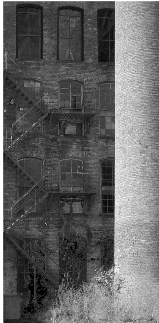
S EMPIRE ST GARMENT FACTORY WILKES BARRE, PA 20 FOOT INTERIOR BAYS
