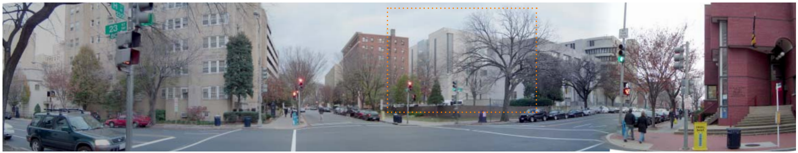
VIEW OF SITE FROM THE CORNER OF 23RD STREET NW AND H ST NW LOOKING SOUTHEAST
