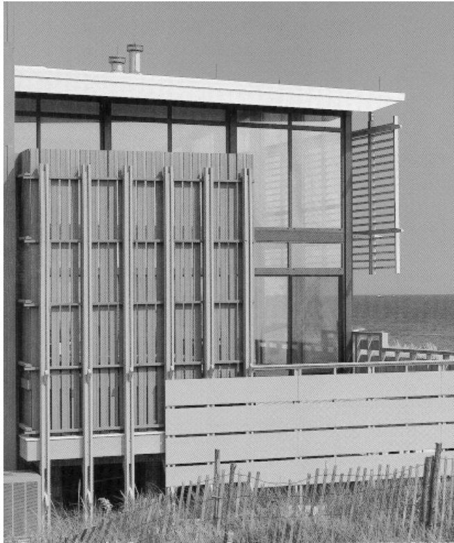
New Jersey Beach House (1999) by Brian Healy and Michael Ryan. The gridded wooden louvers provide sunshading and privacy while maintaining the ocean view. They also function as window protection for the large expanses of glass in case of severe storms.
