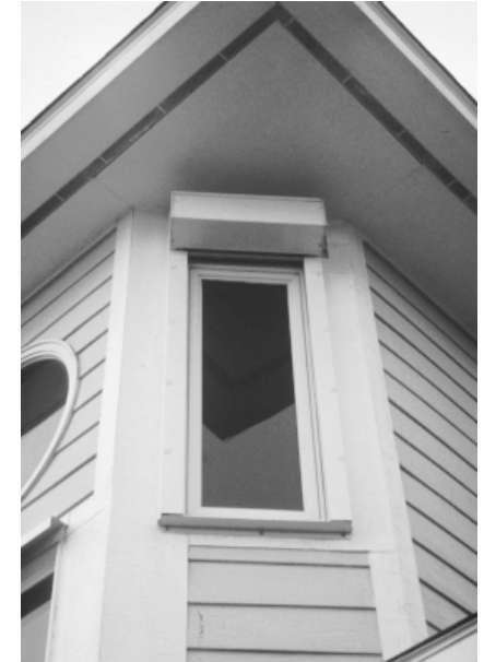
Metal roll-up shutters operated from inside allow this second floor window to be quickly and easily protected.
