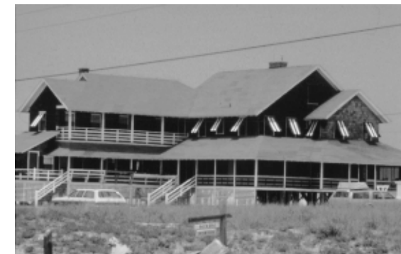
A bed and breakfast in Nags Head. Built on the ocean in 1932, it was moved across the beach road in the 1980's to avoid the encroaching seawater.
