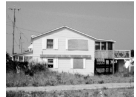
Nailed on plywood sheets are dangerous to install, damage the building envelope, and often blow off to become wind-borne projectiles themselves.
