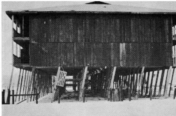
A house with insufficient lateral bracing after a hurricane. The shear walls have protected the interior, but a lack of bracing below flood level caused major damage to the piles.
