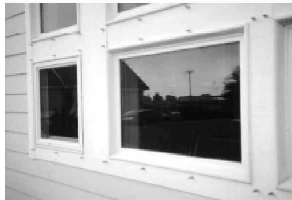
These exposed bolts are ready to accept pre-cut pieces of plywood that can be quickly placed and secured without damaging the windows or trim.
