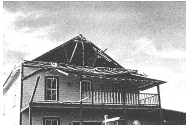
A gable end blown out by Hurricane Andrew. When a building envelope is breached by high winds or projectiles, internal pressurization can “pop” out wall or gable ends that are not properly connected. While the structural damage to this house is minimal, the ensuing water damage rendered the house a complete loss.
