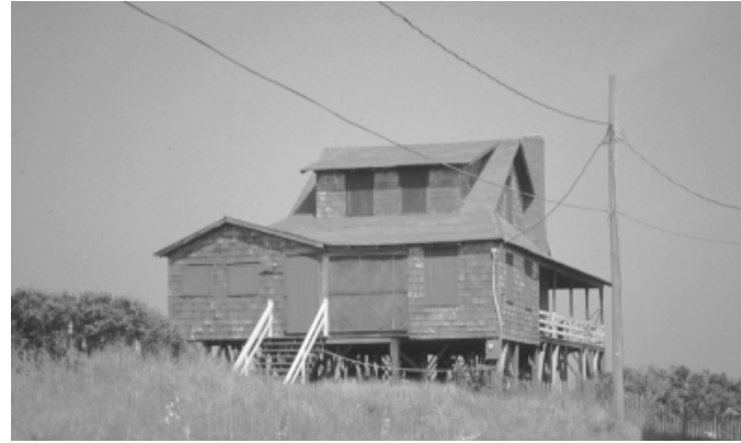
The wooden storm shutters on this house are closed during the off-season to provide protection from both the elements and thieves.
