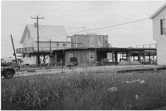
All that remains of a house in Louisiana after Hurricane Andrew. The connection between the foundation and walls was obviously inadequate as the upper floor and roof of this house were found over 150 feet down wind.
