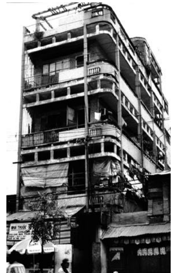
Existing: Typical housing style in CanTho
