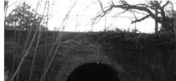
Existing tunnel condition
