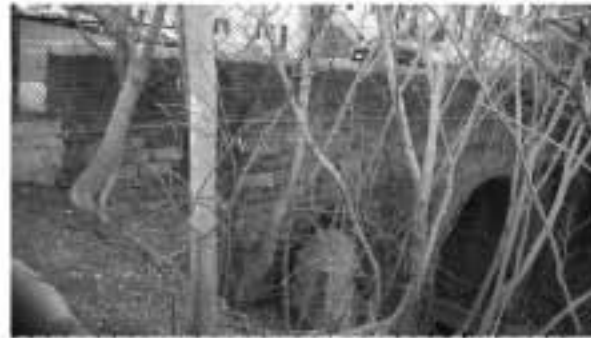
Existing tunnel condition
