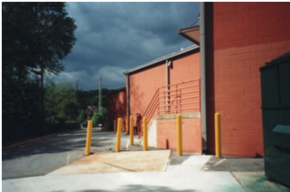
Photo 4.37. Well-hidden waste storage in blind passage.
