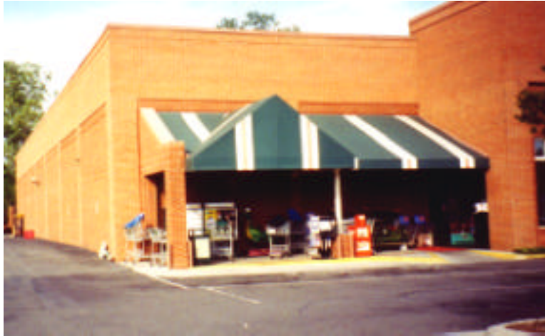
Photo 4.65. A combination similar to that seen in Photo 4.64, but without the seating, occurs at the left entrance.
