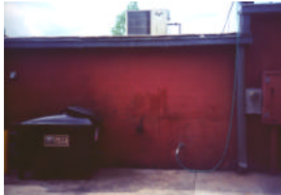
Photo 4.54. Shopping Center rear wall on Kenilworth Avenue, facing a row of residences (see Photos 4.55 and 5.56).
