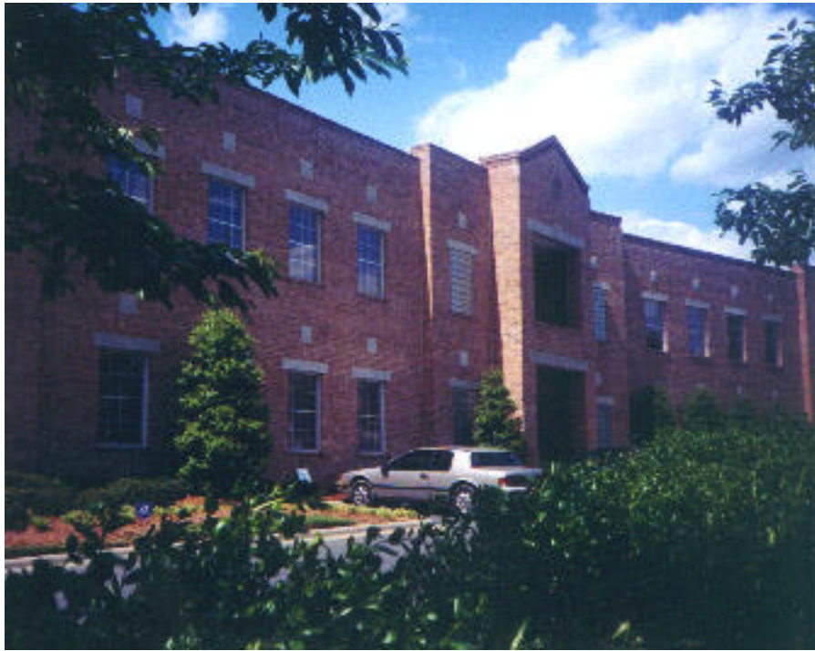
Photo 4.26. Office building across from Dilworth Gardens on Scott Avenue.
