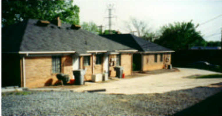
Photo 4.51. Apartments adjacent to Center back, Kenilworth Avenue.
