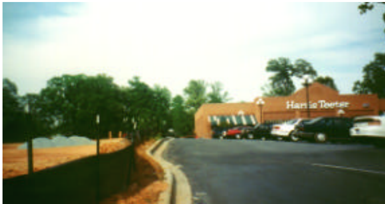
Photo 4.58. Construction to the Center's left, on new land acquisition.
