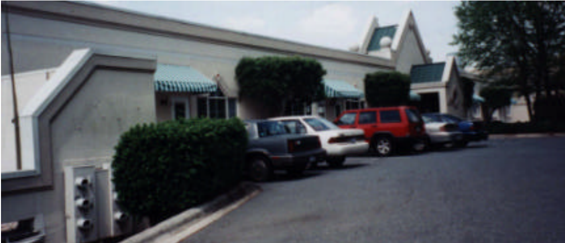
Photo 4.11. Second story rear entrances: Massing of landscape materials forms an instantly legible pattern, together with canopies and double gables at stairway, identifying entrances and pathways.
