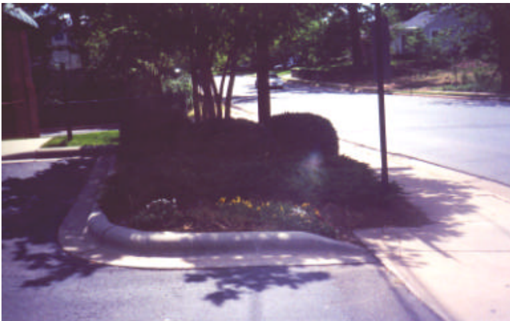
Photo 4.33. Scott Avenue entrance to Dilworth Gardens. Sidewalk ends here.
