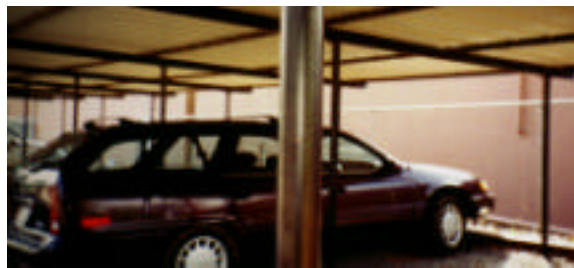
Photo 4.52. Apartment parking at Center back wall.
