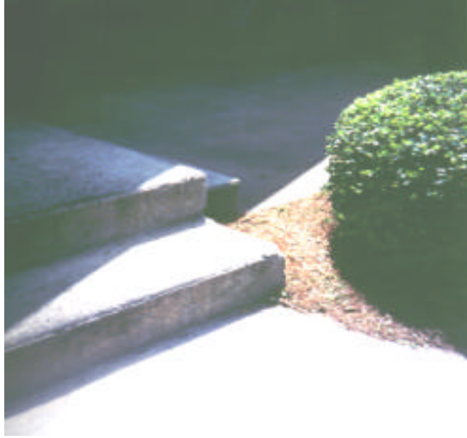
Photo 4.22. Awkward stair and landscaping configuration.
