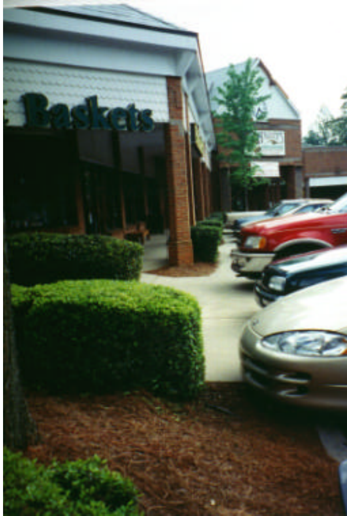
Photo 4.41. Internal pathways unclear due to confusing pavement and landscape elements.
