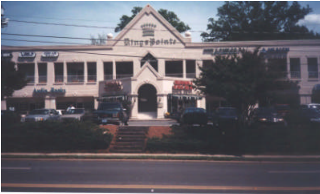
Photo 4.14. Flight of stairs from South Kings Drive sidewalk. Not even paint striping protects pedestrians when crossing the parking lot to the main entrance and sidewalk.
