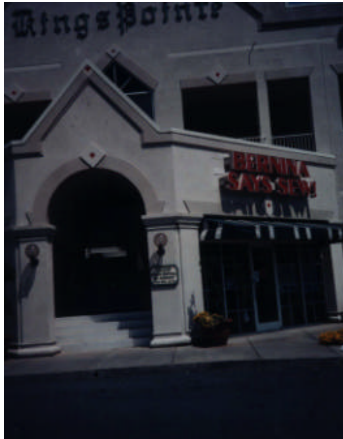
Photo 4.7. KingsPointe stair entrance at ground level.
