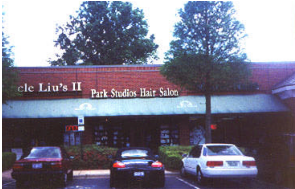
Photo 4.23. Unarticulated building facades impede wayfinding.
