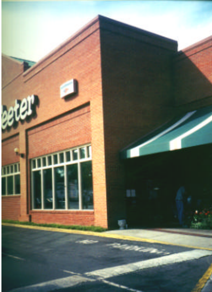
Photo 4.46. An example of complex details well carried out (note windows and brickwork).
