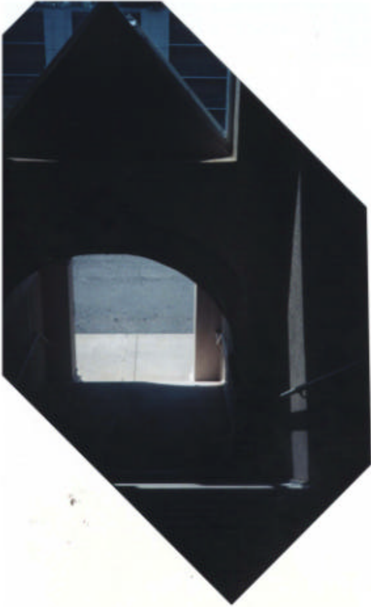
Photo 4.8. Stair view from upper to lower level at KingsPointe.
