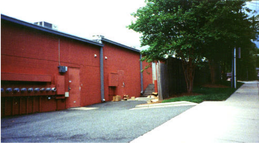
Photo 4.20. Landscaping screens portion of waste storage at Center back.
