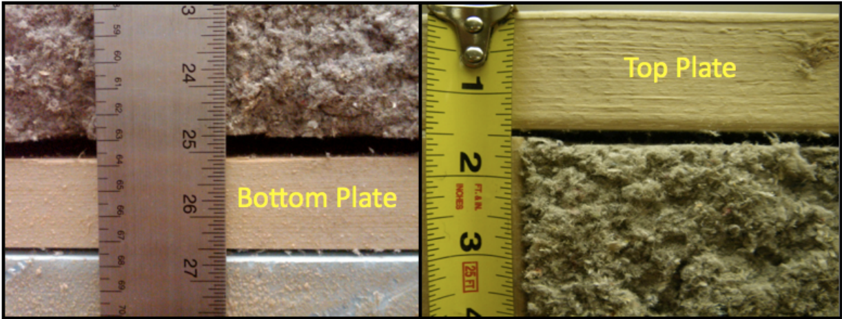
Figure 6-1: Picture depicting the spray-applied cellulose settling and shrinking, which created a gap between the insulation and wood framing.
