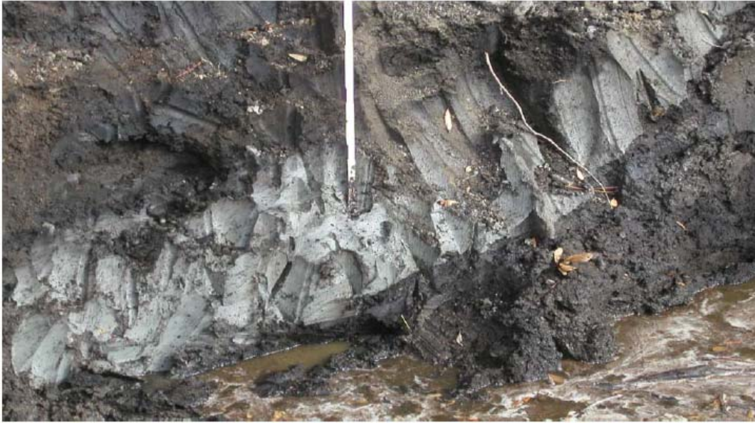
Figure 18: Exposed failure plane with a marsh layer between two clay layers (IPET 2007)
