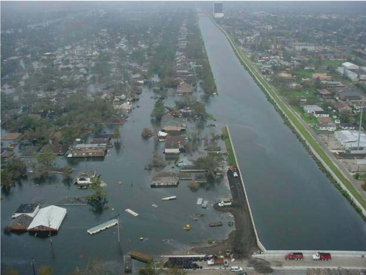
Figure 10: Aerial view of breach in floodwall on east side of 17 th Street Outfall Canal (IPET 2007)
