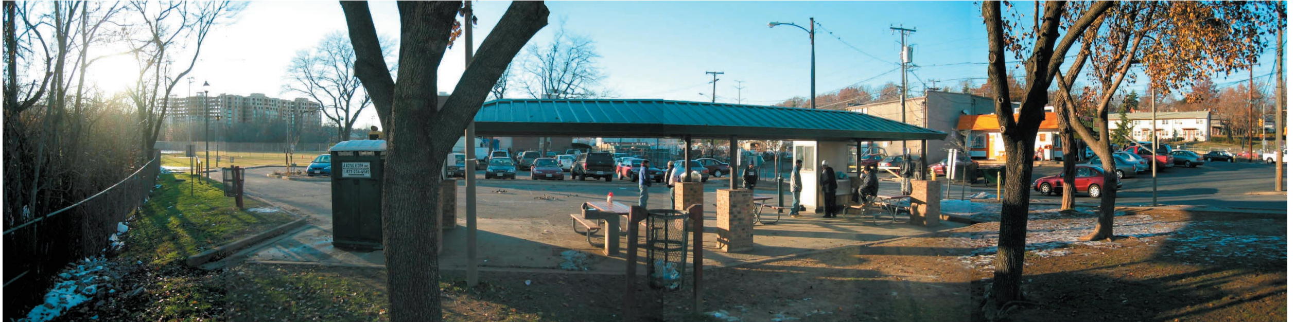
Fig. 2.4 - Photo of the SEEC day labor site and pavilion structure.
