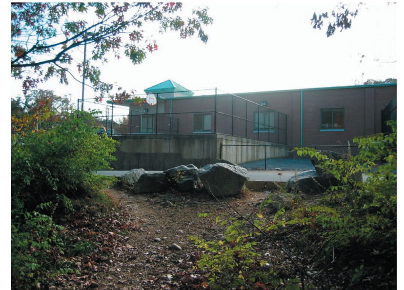
Fig. 4.1. Boulders block access to the only connection between the AMCC site and the existing trail along Four Mile Run.
