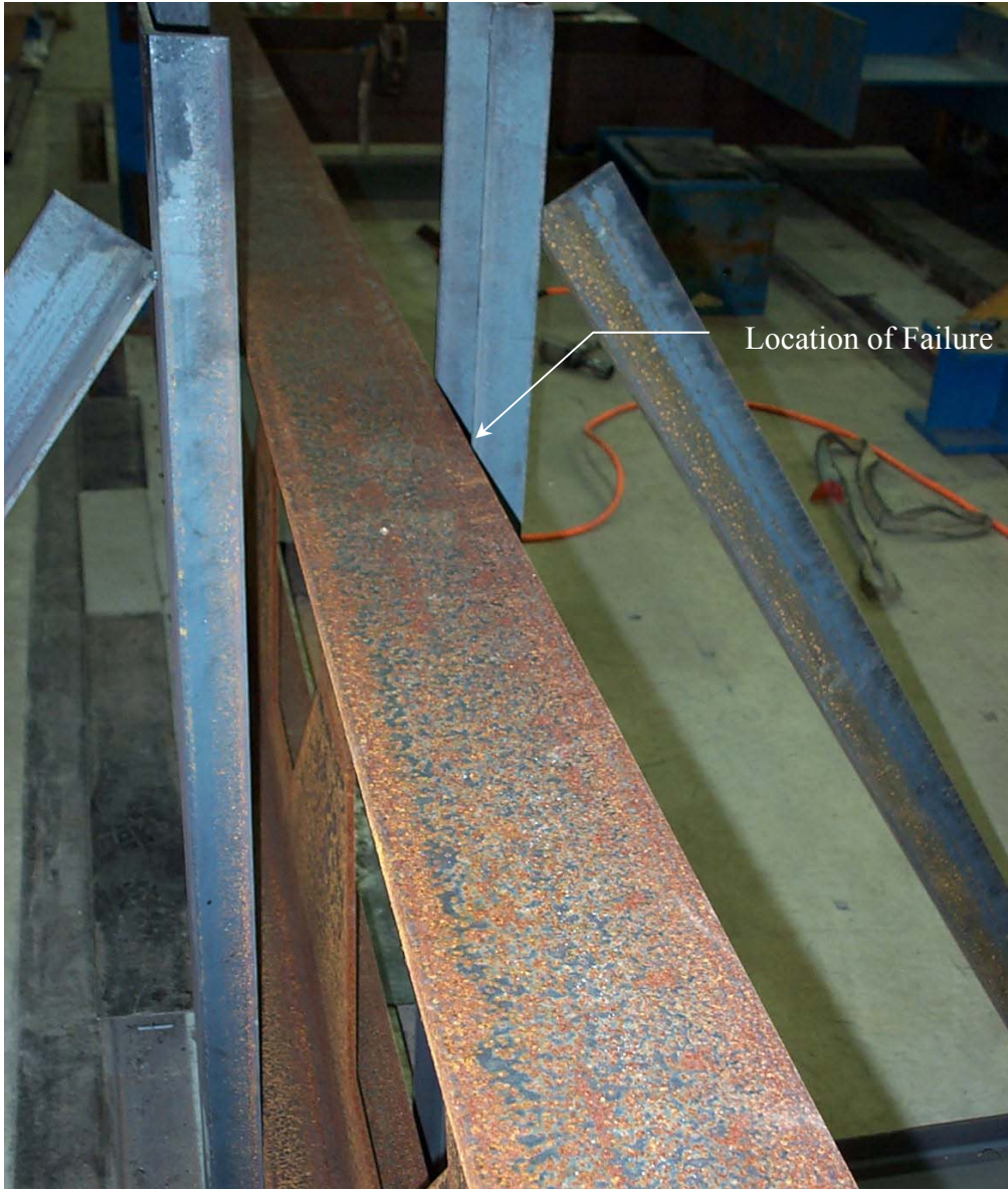
Photo of CB27x40 Specimen at failure
