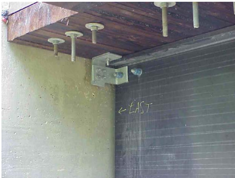
Figure 7.8: End Constraints
