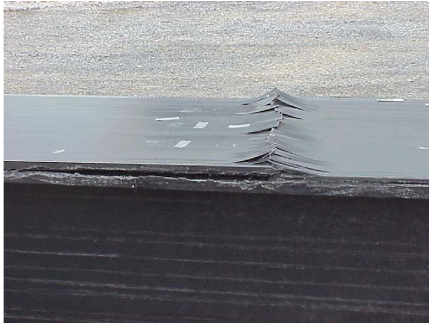
Figure 1.5: Close-up of a Failed Section
