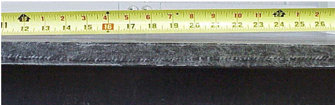
Figure 7.5: Flange Surface Irregularities
