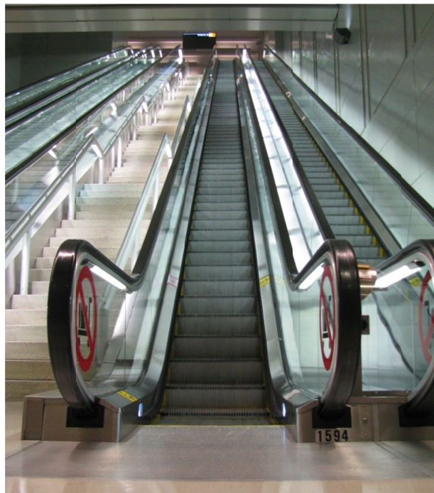
Figure 2.2: Escalator with Glass Handrail Balustrades, Dulles International Airport
