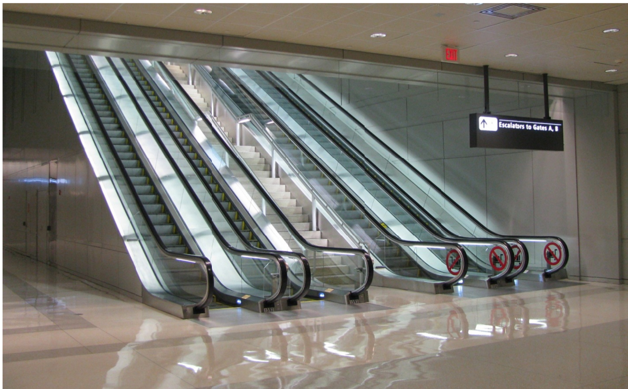
Figure 1.1: Typical Escalator Bank, Dulles International Airport
