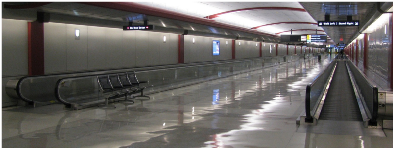
Figure 1.2: Typical Moving Walkway Installation, Dulles International Airport
