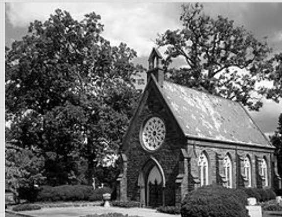
Chapel built by James Renwick on grounds of the Oak Hill Cemetery.
