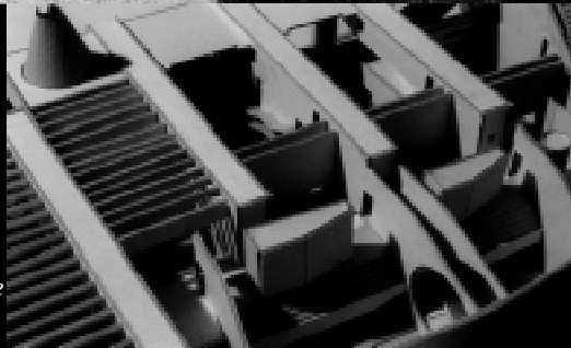
The walls connected by the ‘beam-galleries’
