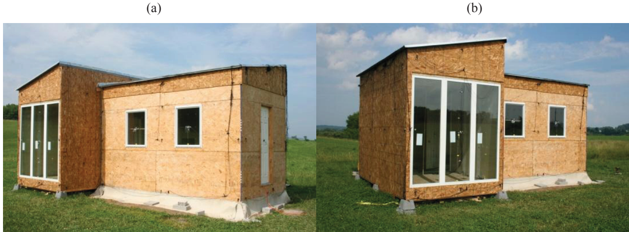
Figure 3.20: Pictures of the two room structure showing (a) the original structure and (b) the addition structure.
