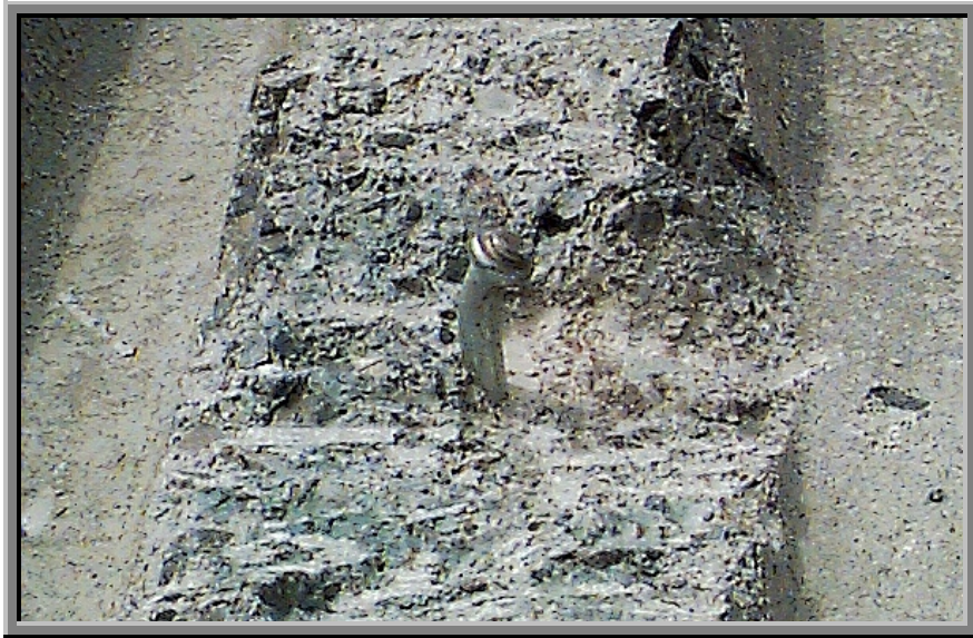
Figure 3.4 Typical Screw Shear Failure (Note: concrete removed to provide clear view of sheared screw)
