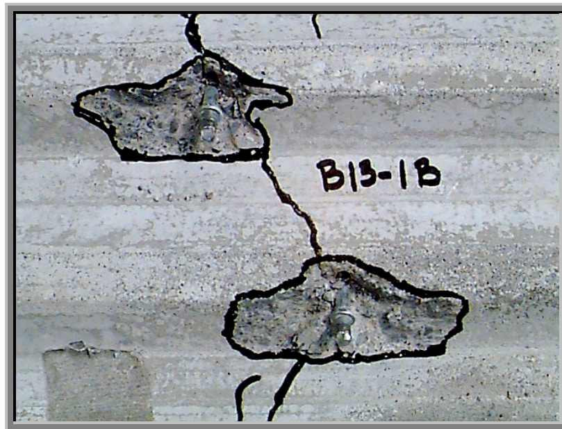
Figure 3.7 Typical Rib Failure Observed in Series B Tests
