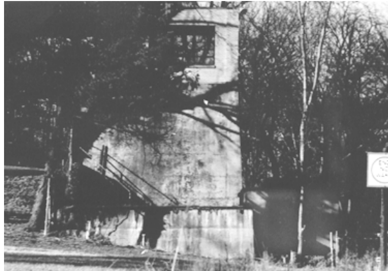
Water processing plant
