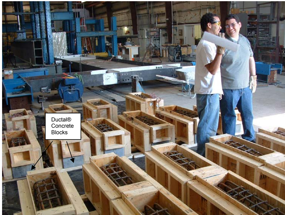
Figure 3.12 Lightweight concrete formwork
