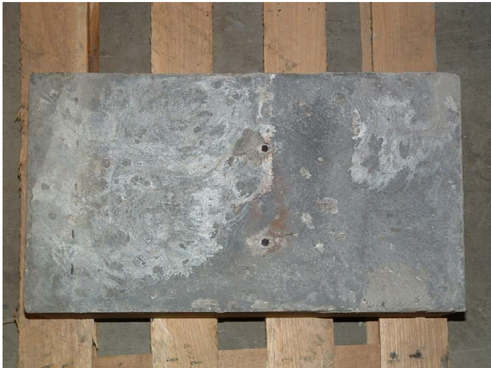
Figure 4.17 Undamaged Ductal® Side of Double Leg Specimen (After Testing)
