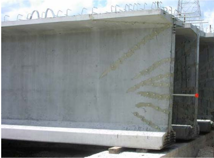
Figure 1-2. Photo of a repaired 95 in. PCEF bulb-tee girder from Davis, et al. (2005)
