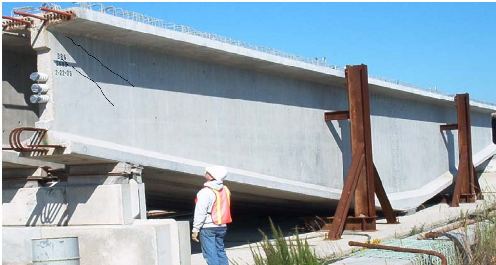
Figure 3-7. Anchorage zone cracking observed in deep haunched girders
