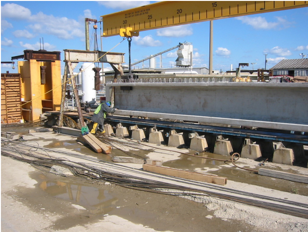
Figure 4-9. Test girder lifted from casting bed on October 25, 2006
