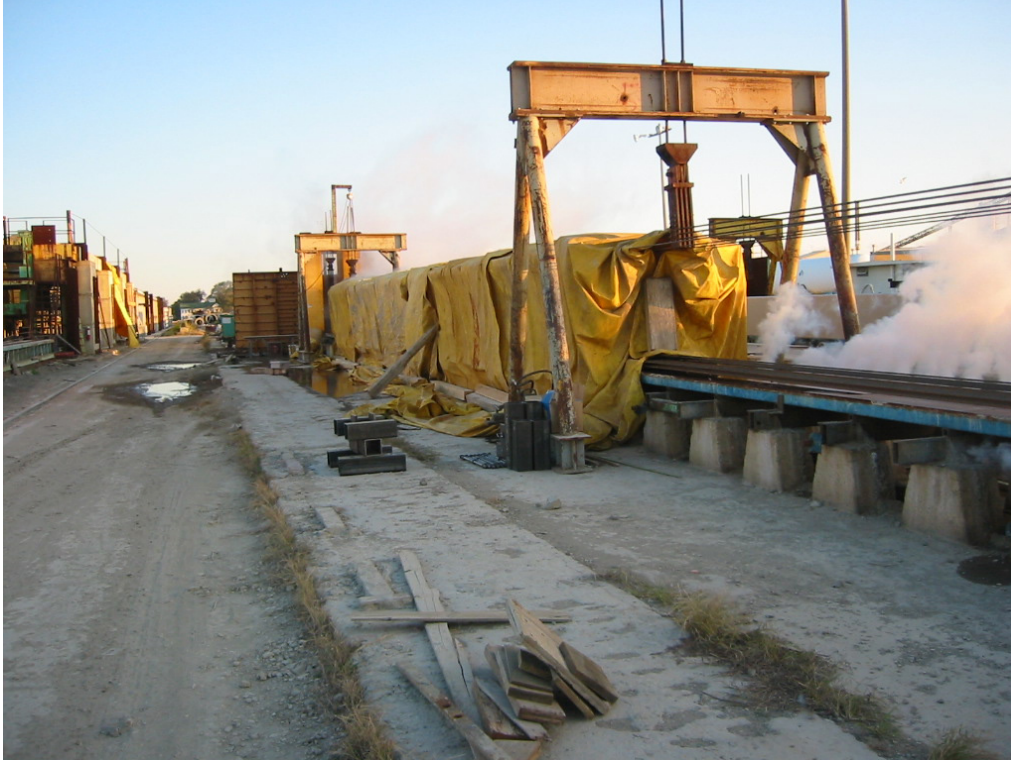
Figure 4-8. Girder steam curing on October 25, 2006
