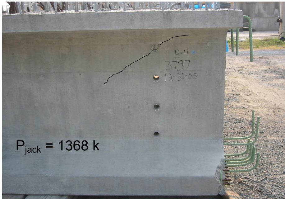
Figure 3-1. PCBT-53 anchorage zone case study – fair condition
