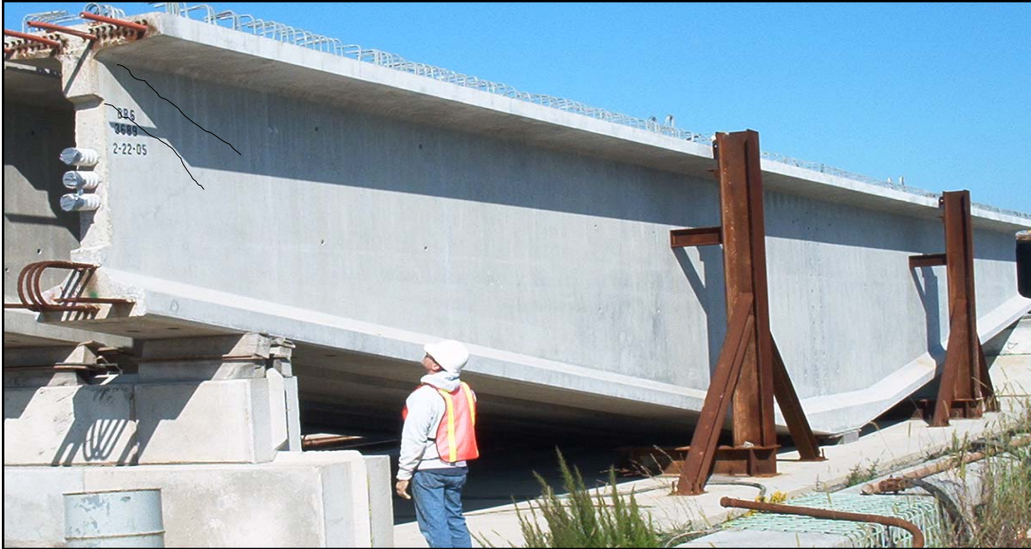
Figure 1-3. End cracking in a splice girder pier segment
