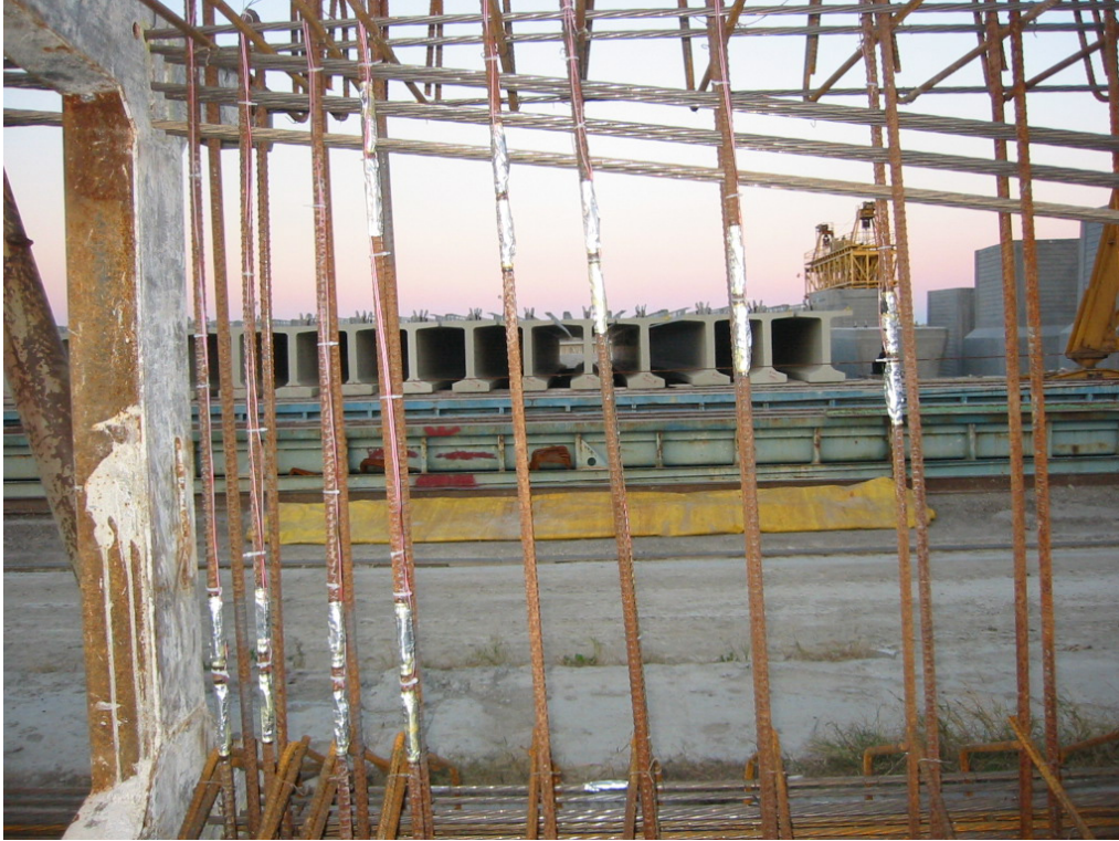
Figure 4-6. Strain gages installed at the 18 ksi anchorage zone
