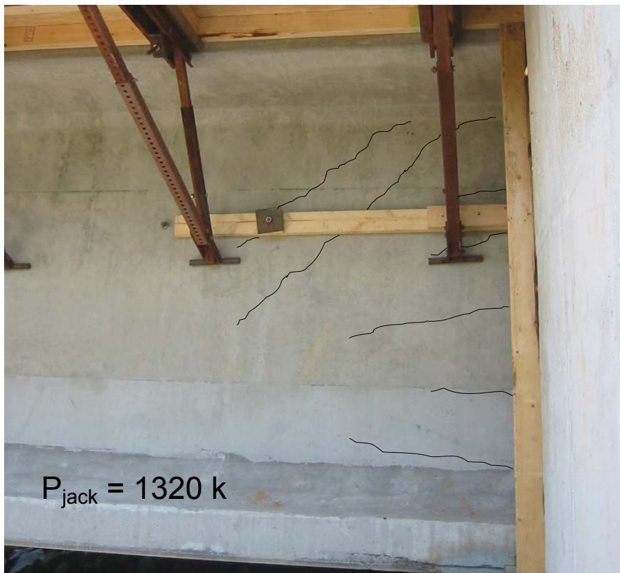
Figure 3-4. PCBT-77 anchorage zone – poor condition
