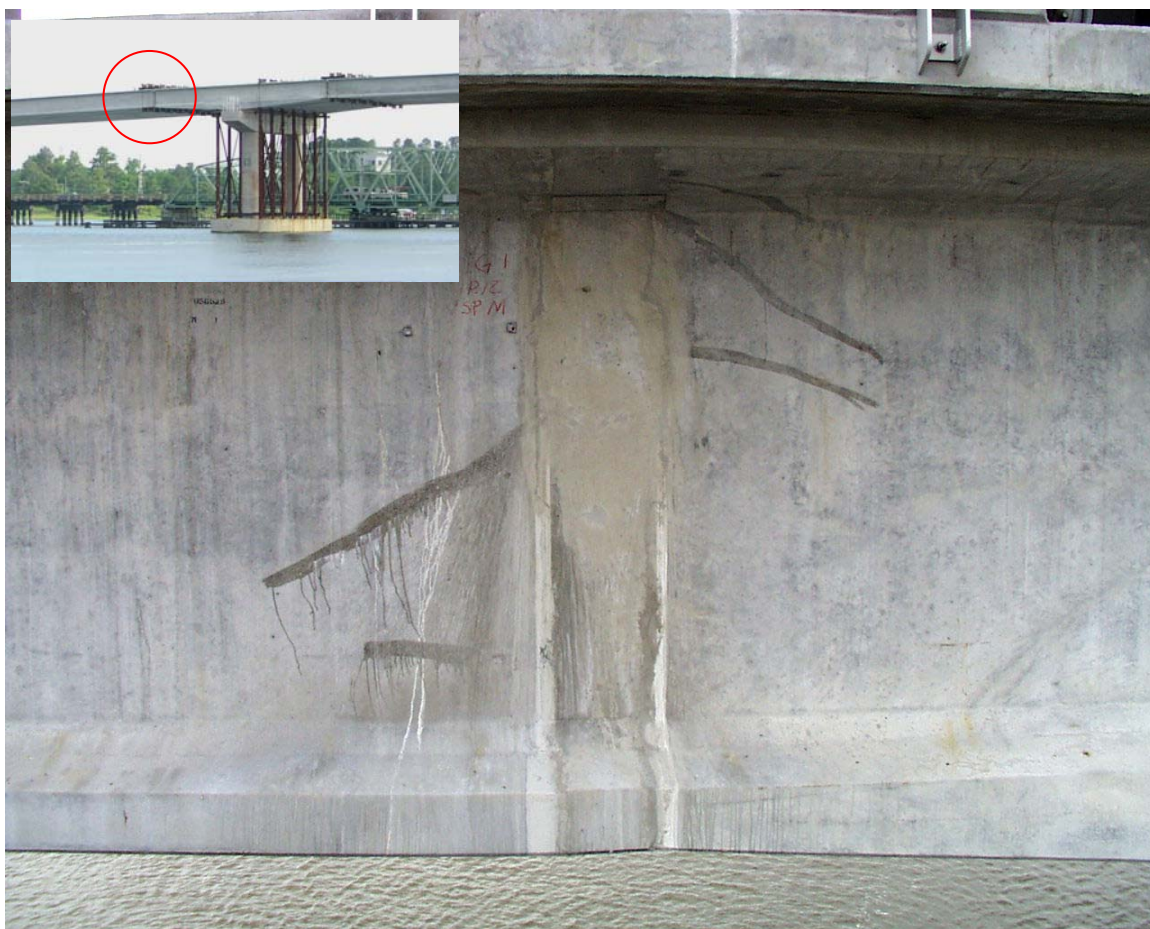
Figure 3-8. Anchorage zone cracking of in-service haunched girder and “drop-in” girder (photograph by Rodney T. Davis)
