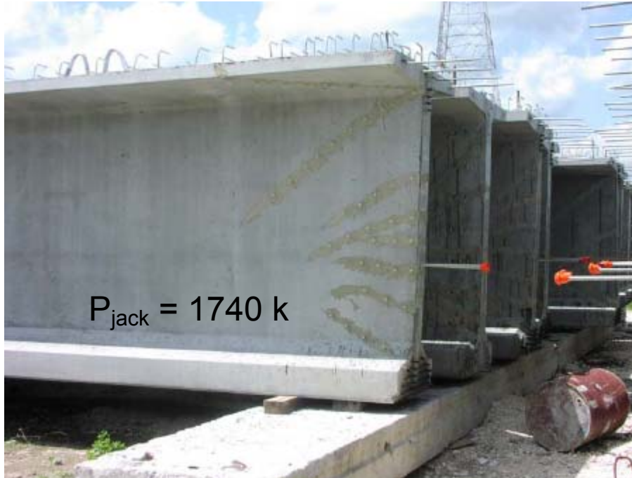
Figure 3-5. 95.5 in. PBCT beam ends with repairs. Photograph from Davis, et al. (2005)
