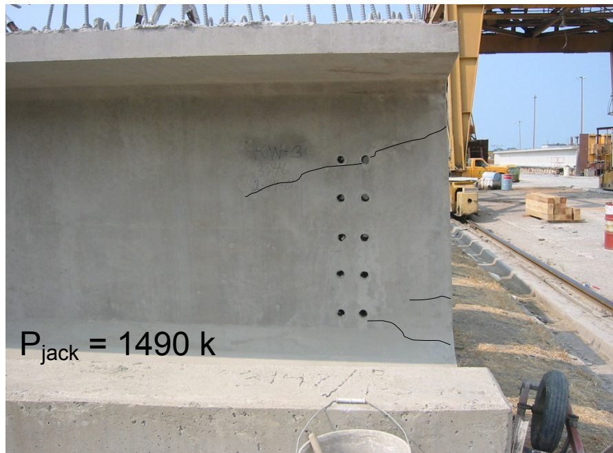
Figure 3-2. PCBT-61 anchorage zone case study – fair condition
