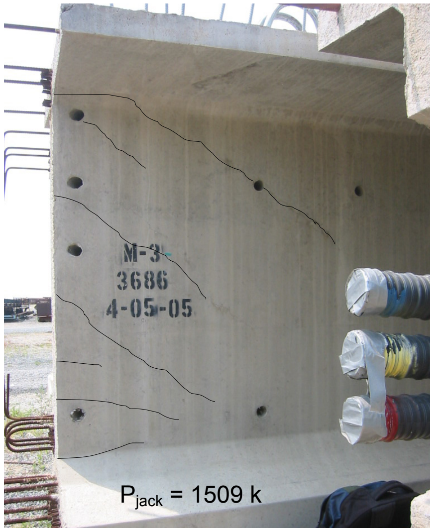
Figure 3-3. PCBT-77 anchorage zone case study – poor condition
