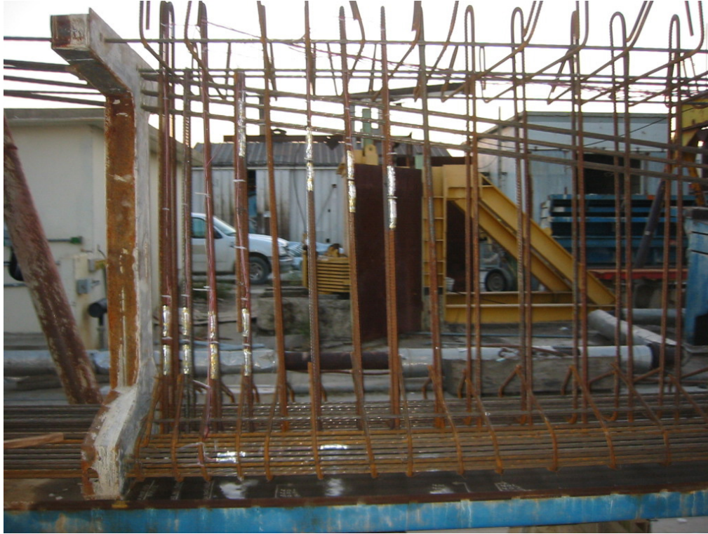
Figure 4-5. Strain gages installed at the 12 ksi anchorage zone
