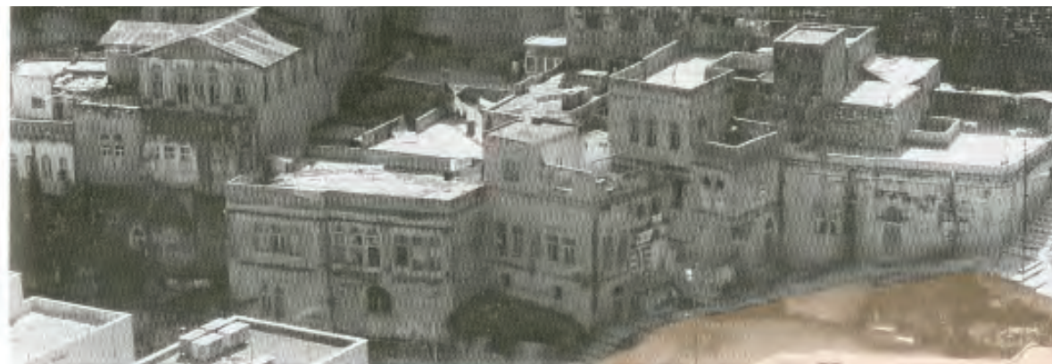
Photograph of historic complex taken from the top of previously existing police station
