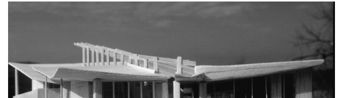
Details of the atrium roof, The High School Project.
