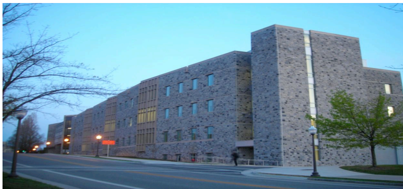
Figure 3-2-4-9-2a View of the ICTAS building (Photo by author, 2008)
