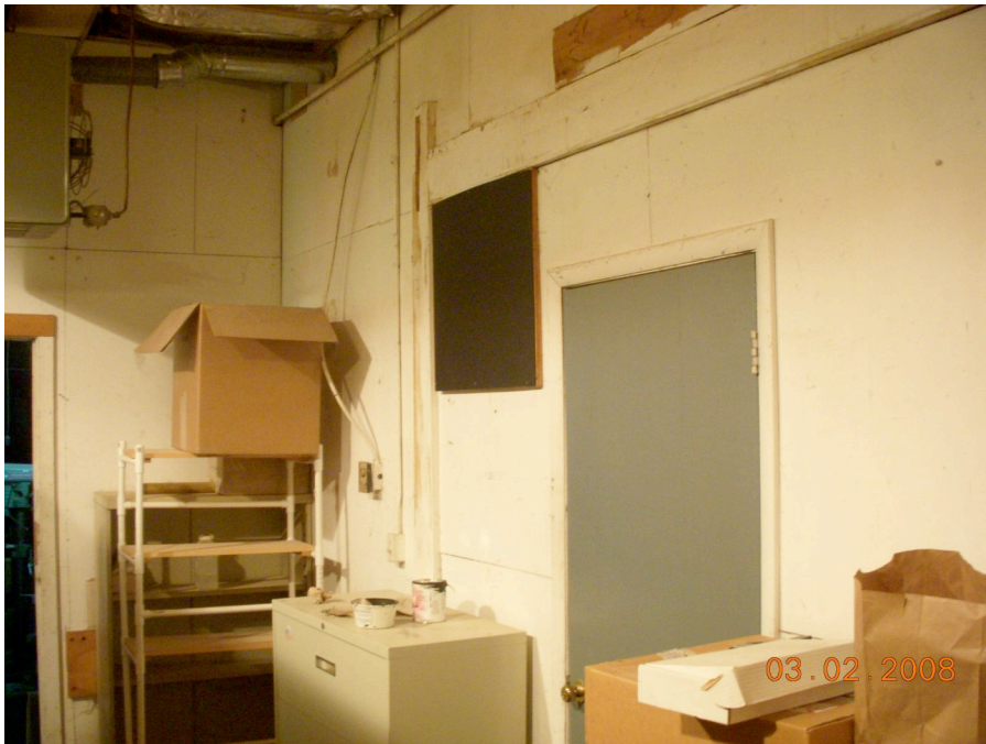
Figure 3-1-1b Picture of “Blocked” window (Photo by author, 2008)
