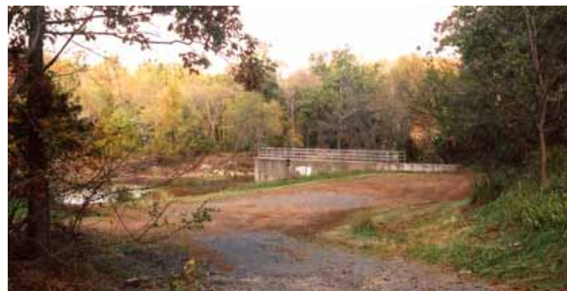
Existing conditions at Fishway location.
