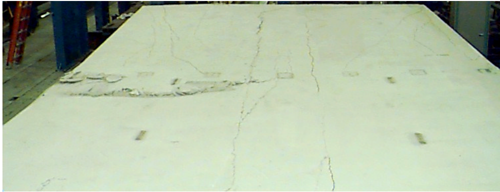
Figure 3.64 West End Slab Cracking (H-2)
