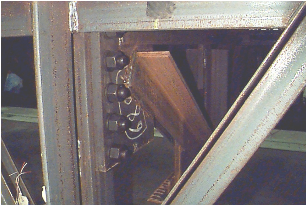
Figure 2.15 Bolted Connection Detail (FF-1,FF-2)
