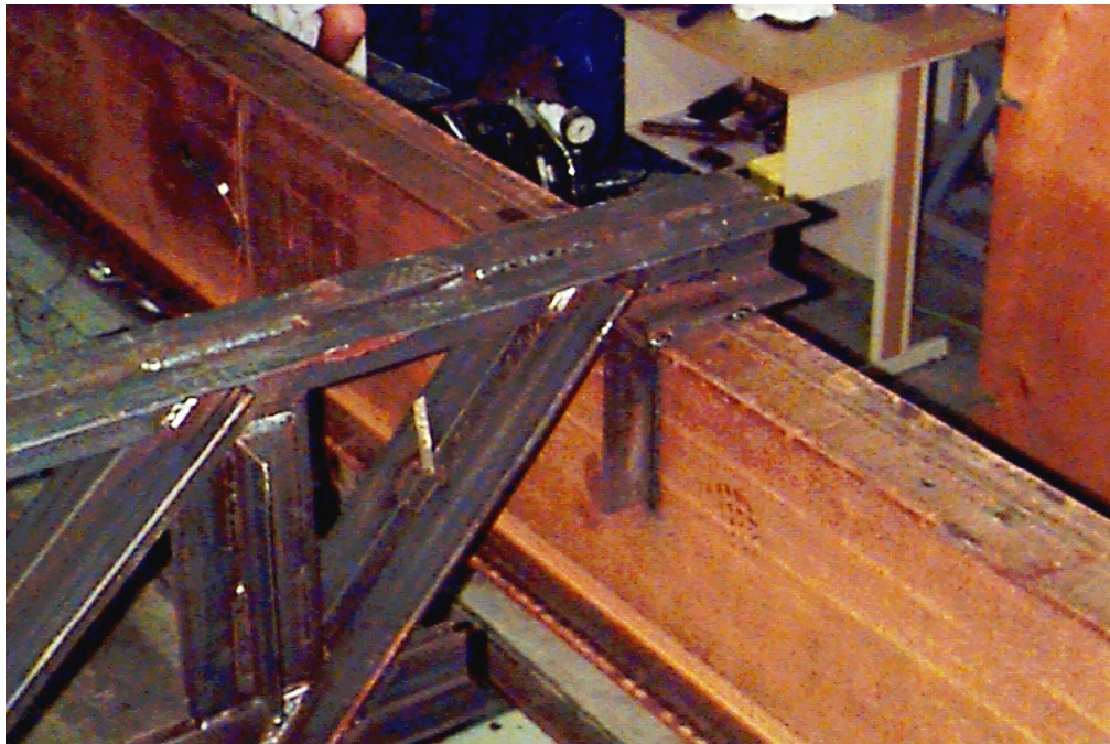
Figure 2.16 Joist Bearing Detail (H-1, H-2)
