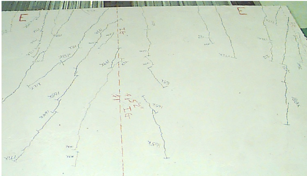
Figure 3.59 East End Slab Cracking Over EG/IG (FF-2)
