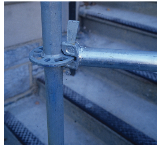
Standard scaffolding connection
