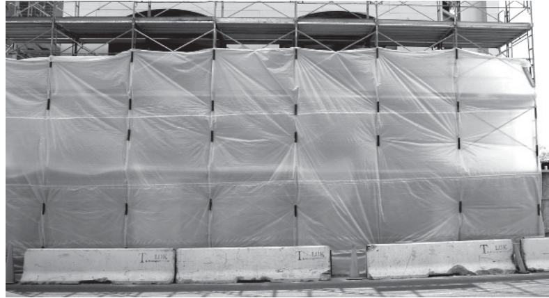
Building under construction with tarps moving in the wind.
