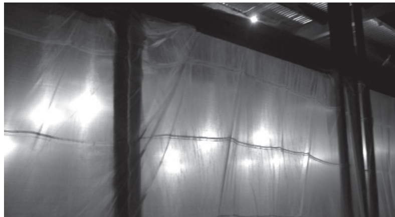
Building under construction at night with transparent tarps illuminated from the inside by electric lights.
