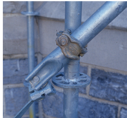
Irregular scaffolding connection
