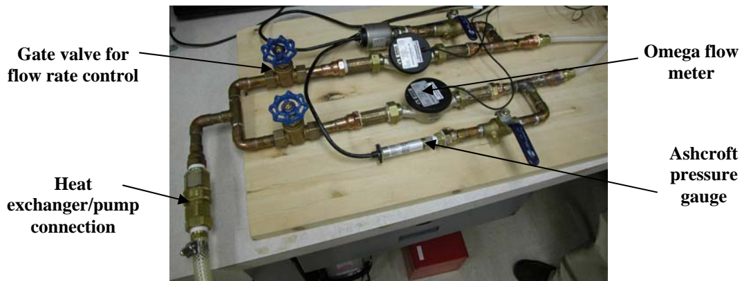
Figure 3.30 Fluid measurement and control system
