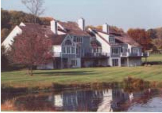
Figure 13 Rear view of townhouse units and ponds.
