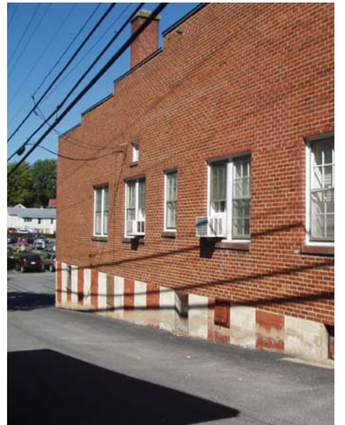
The long sides of the building are irregularly punctured by windows. Long brick walls deteriorate through spalling, efflorescence and crumbling mortar. Cooling units and an abandoned flue reveal the methods to heat and cool the building.
