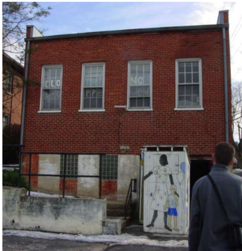
For approximately 50 years an addition sat behind the building which served as a jail, and covered parking garage for the fire department. The addition was removed in the 1980's to make six parking stalls. The rear face of the building now hosts a drop box for a clothing bank which operates upstairs.
