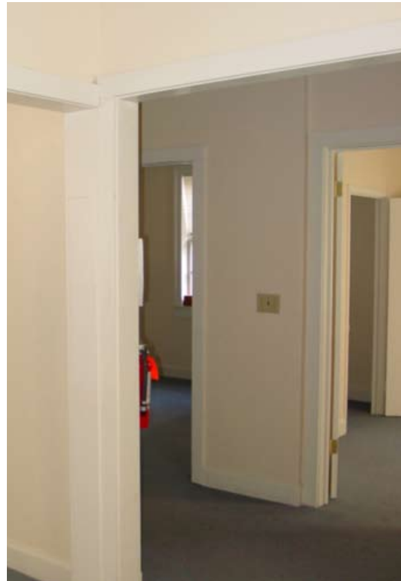
There are several layers of change evident in the many non-load-bearing partitions within the Church street level. A central hallway connects rooms and open areas of varying sizes.
