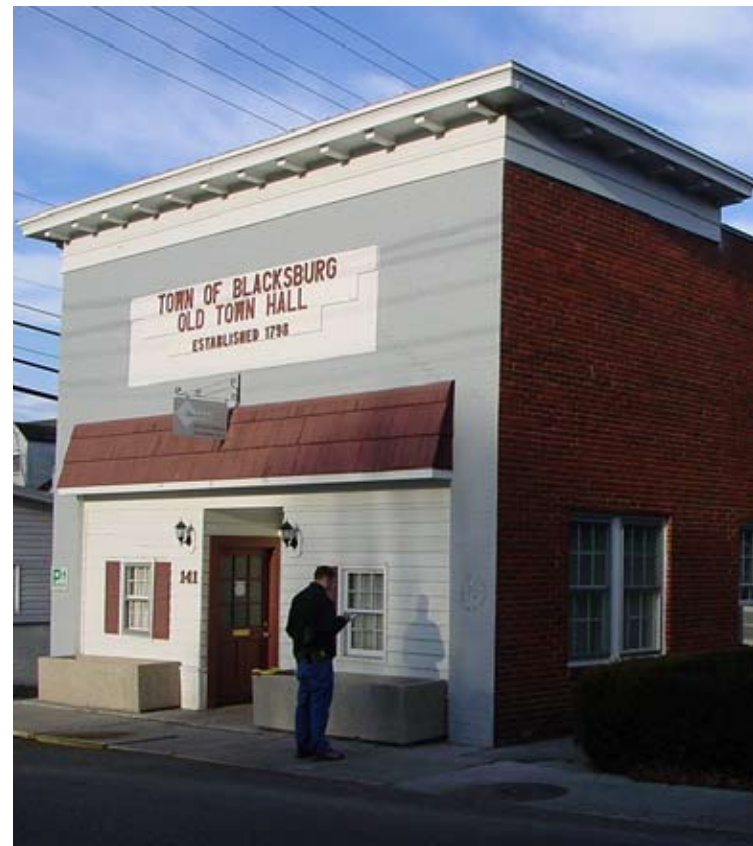
The rebuilt facade is based on the original glass and wood storefront. It was filled in after the building was struck by a car in the mid 1980's. Two planters resting under the narrow wood canopy are designed to withstand a car impact of 15 mph.
