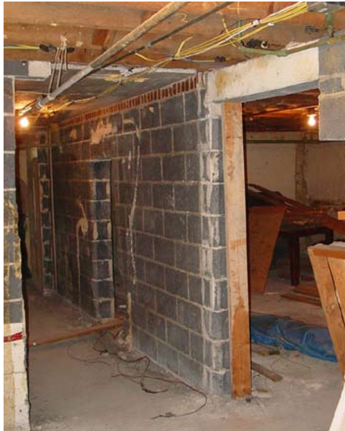
The parking lot level of the building stands as a maze of both wood and concrete block bearing and non-bearing partitions, and a network of pipes and abandoned wiring. The town used it for municipal storage.
