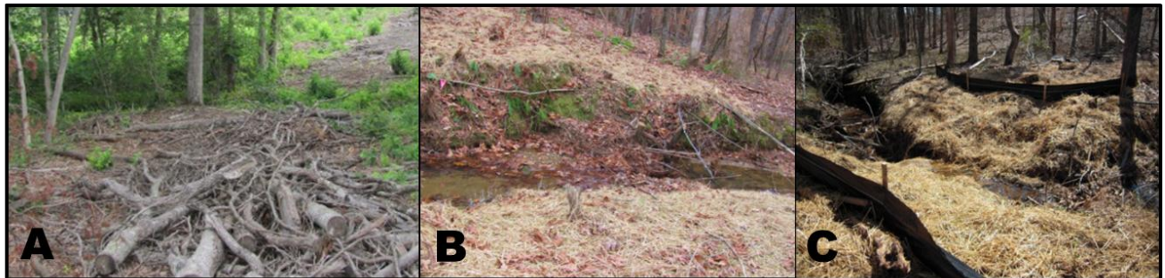
Figure 2. Representative stream crossing approaches that were closed with slash treatments (a), mulch treatments (b), and mulch + silt fence treatments (c).
