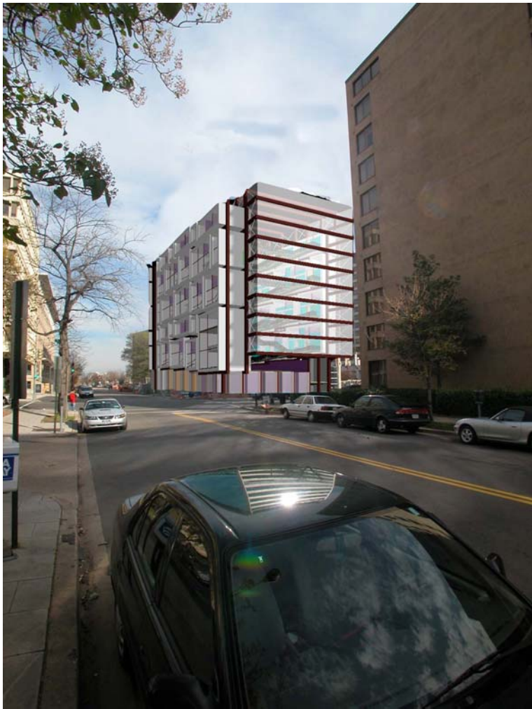
View from the Southwest
