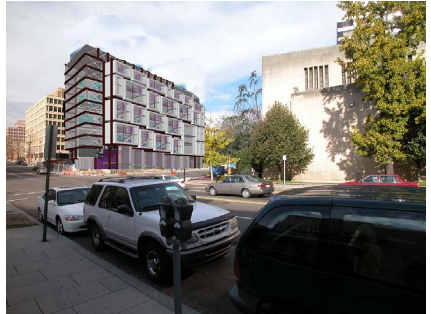
View from the Southeast
