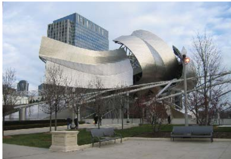
Figure 53. The curving stainless steel of the Pritzker Pavilion defines another district in the park
