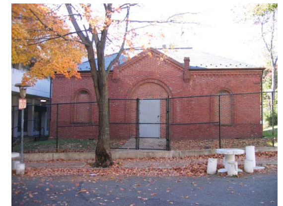
Figure 131. Historic pump house to be reused in recreation area
