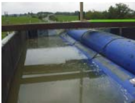
Figure 2-28: Trial 6 at Headwater Elevation of 12 ½-inches
