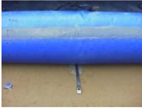
Figure 2-27: Bentonite Cutoff Trench after Tube #2 Installed
