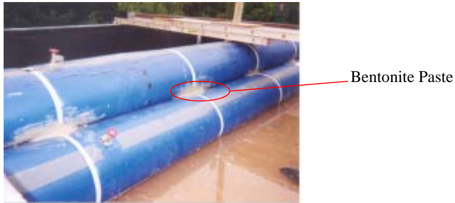
Figure 2-17: Bentonite Paste Applied to Tube #2 and Tube #3 in Trial 3
