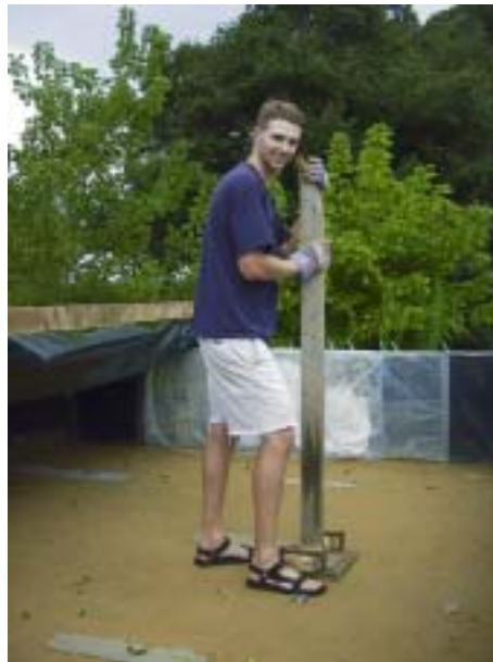
Figure 2-25: Flat Plate Hand Compactor in Operation
