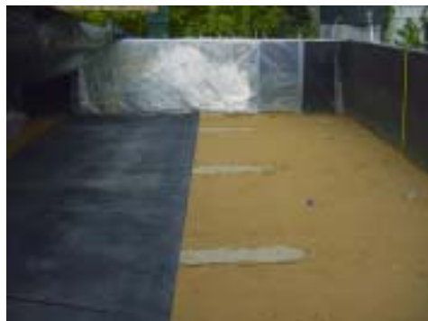
Figure 2-26: Bentonite Cutoff Trenches to Prevent Piping under Strap Locations in Trial 6
