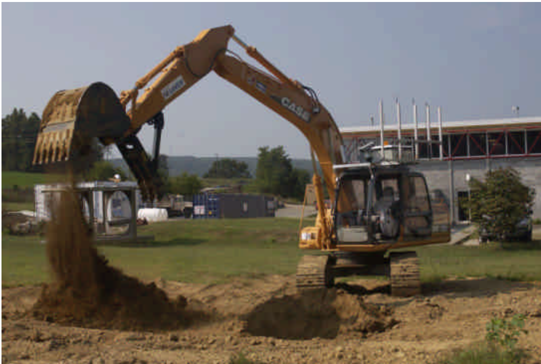
Figure 1-1: Remotely controlled CASE CX160 excavator
