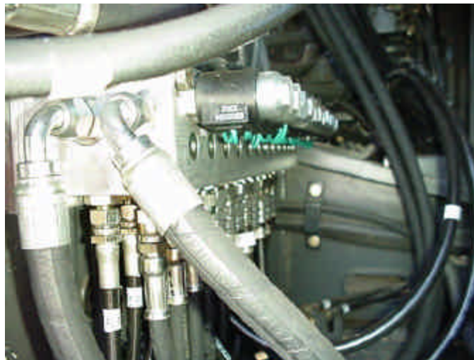
Figure 5-6: Picture of manifold with proportional valves installed
