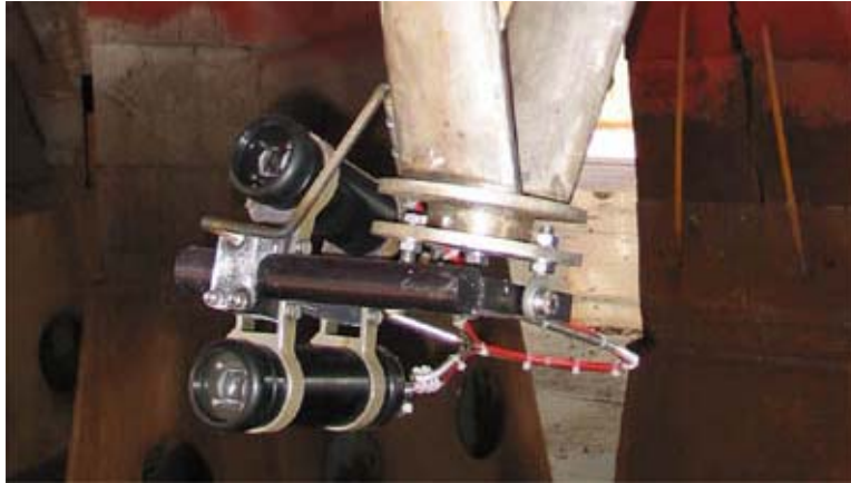
Figure 13 – Installed Laser Probes
