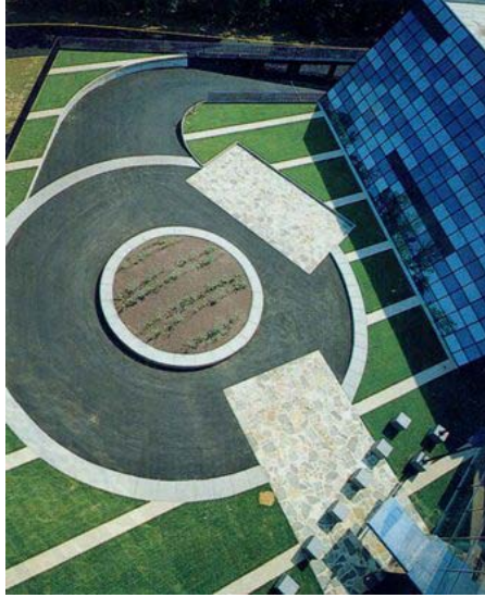
Figure 4.6: Aerial view of the entrance roundabout showing the flagstone “welcome mats”.
