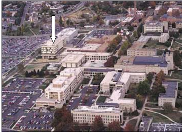
Picture 3.1 Aerial View of Transmitter
