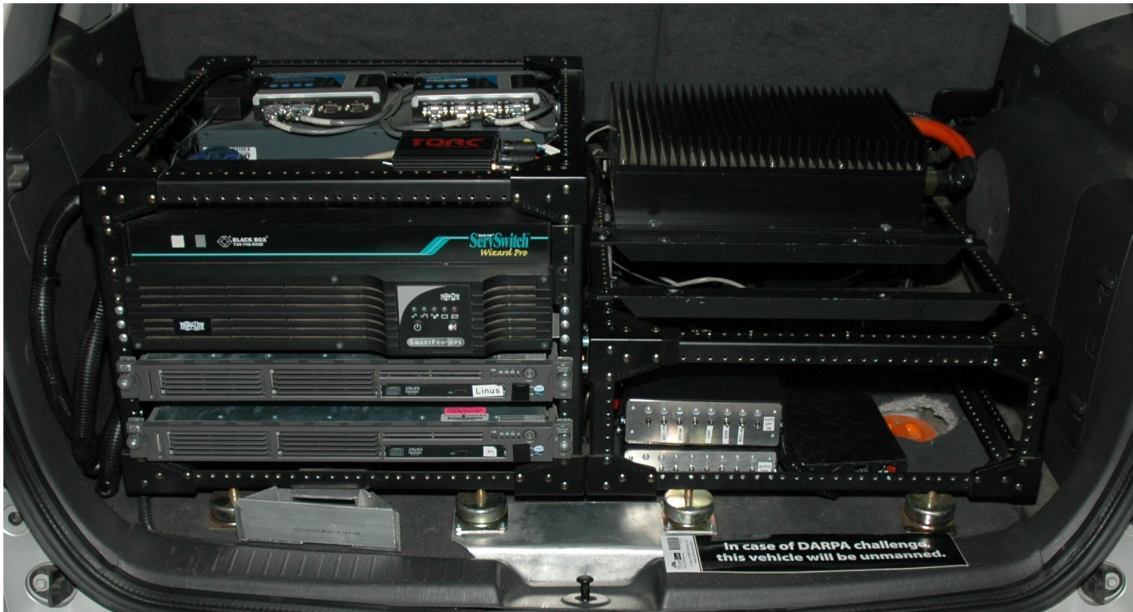
Figure 2.12: Odin's rear rack showing current computing configuration with 2 HP servers.
