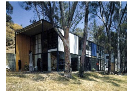
Figure 2.1.1.4 Eames House by Charles and Ray Eames: The Eames house was famously designed to be built from 'off-the-shelf' standardized materials as much as possible (Smith 2007, 23).
