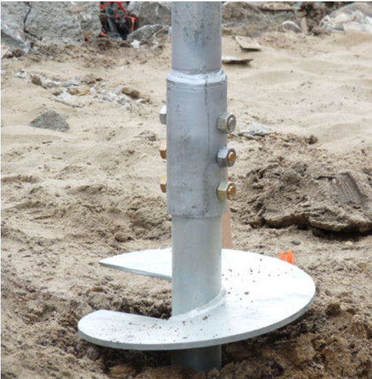
Figure A.8 helical pile (Foundation Supportworks 2012)
