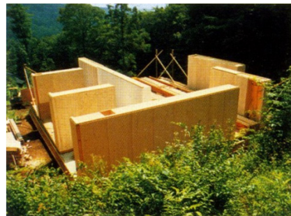
Figure 2.1.1.2 Furniture House by Shigeru Ban: Ban used panelized structures for the interior structural skeleton of the building (McQuaid 2003, 167).
