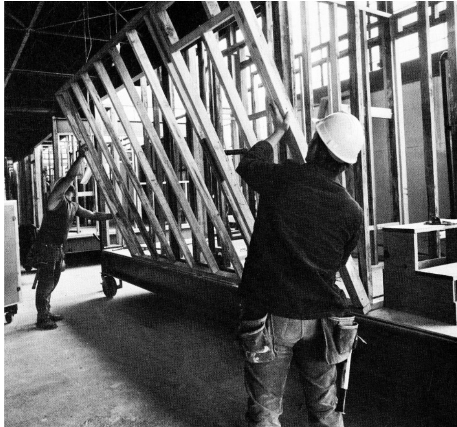
Figure 6.1.2 component assembly line (Reidelbach 1971, 154)
