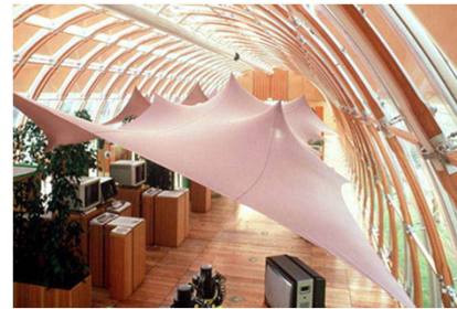
Figure 2.1.1.3 IBM Traveling Pavilion by Renzo Piano: This was a moving exhibition that was broken down into a series of prefabricated components that were designed with demountability and reassembly in mind (Dini 1984, 79).
