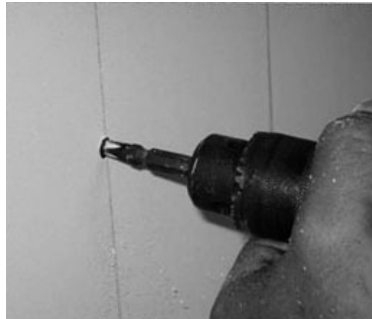
Figure A.18 Magnum Board building product used in place of gyp board (Magnum Building Products 2012)
