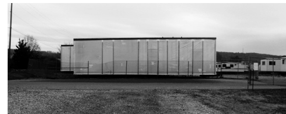
Figure 3.4.1.3: Completed modules are wrapped to protect them from the elements until it is delivered to its final site.
