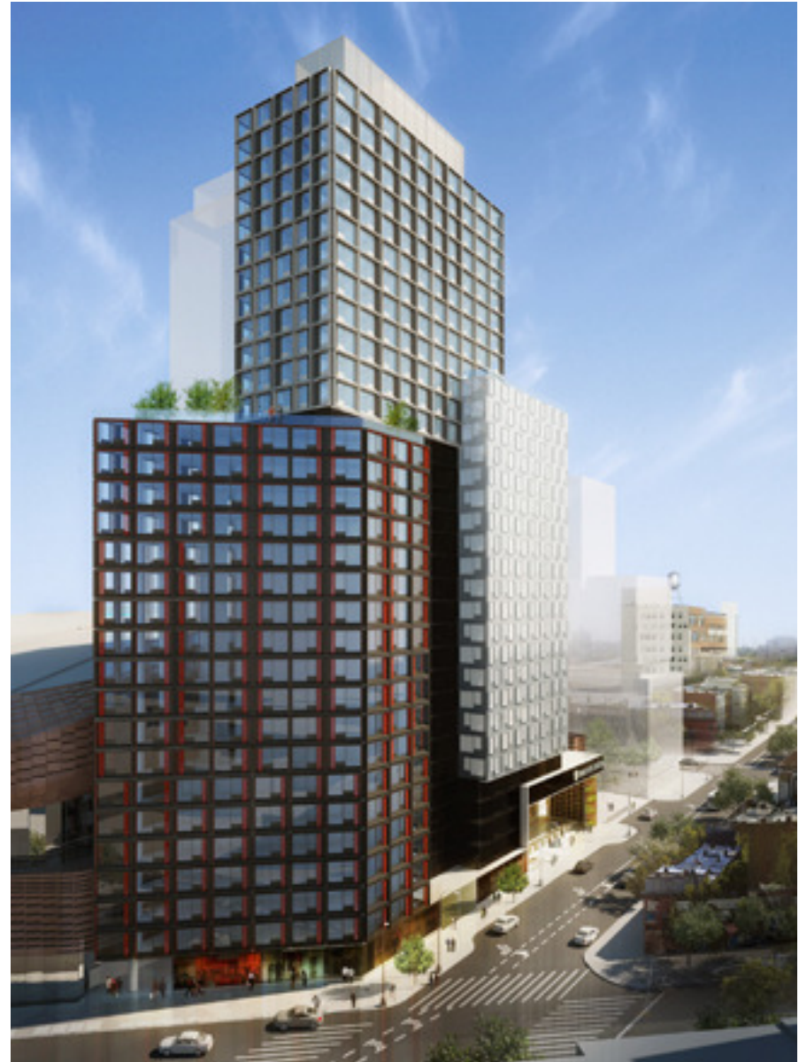
Figure 2.6.5.3 rendering of SHoP Architect's B2 Brooklyn Building for Atlantic Yards: standing at 32 stories, the New York building will be the tallest prefabricated steel structure to date (SHoP Architects).
