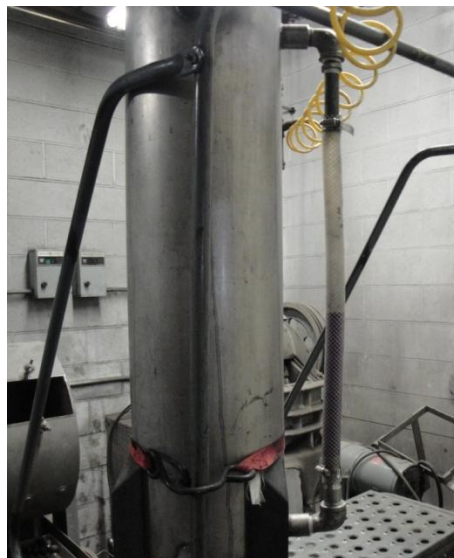
Figure B-10: Fluid level indicator tube on the side of the fluid pressure tank.
