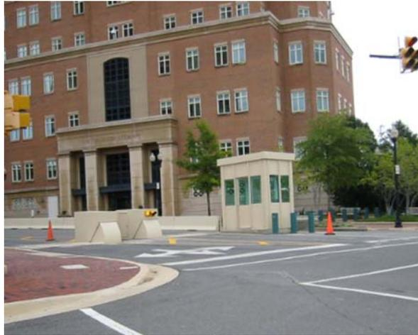
Figure 4, Guard House and delta barriers installed in private street
