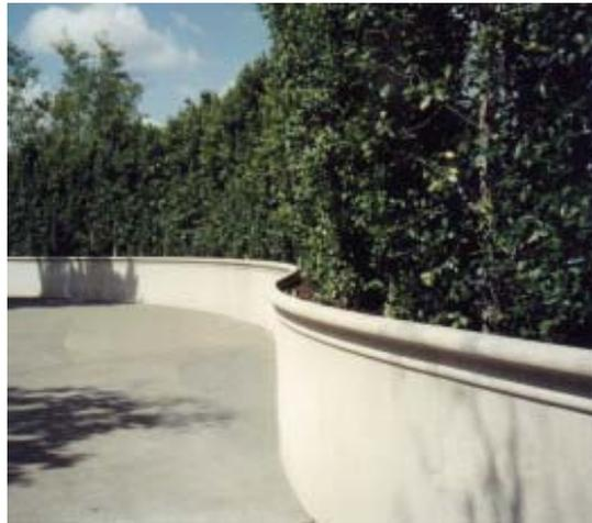
Figure 18, Glass Fiber Reinforced Planter Wall
