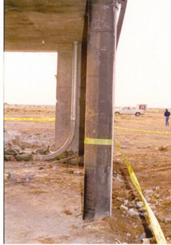
*Ductile response of column ensured by wrapping with carbon fiber reinforced polymer (CFRP)*
