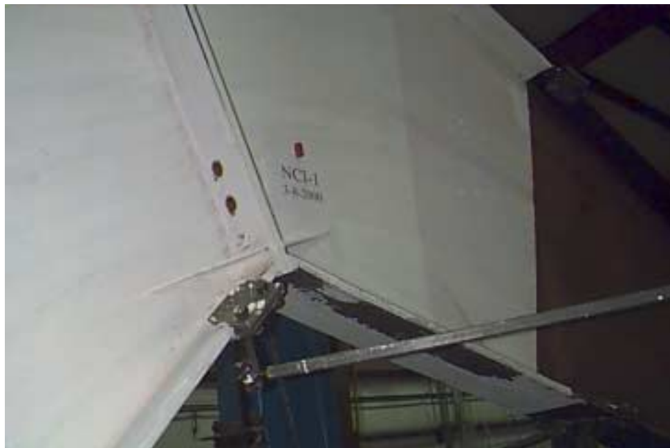
c) Yielding of Rafter Flange
