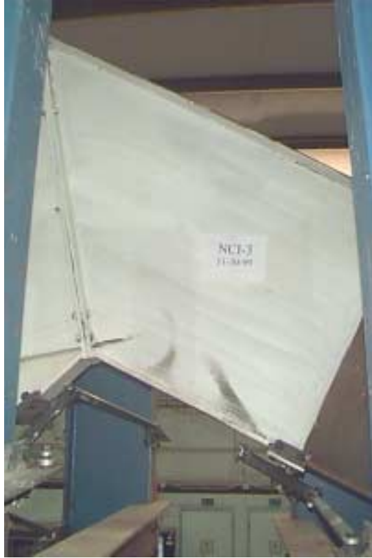
a) Web Buckling of Rafter
