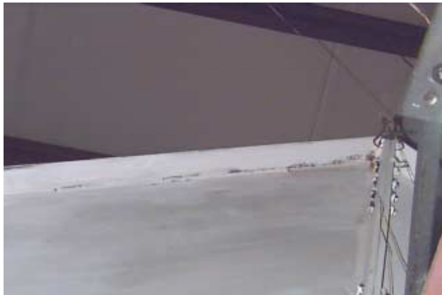
c) Yielding of Rafter Flange
