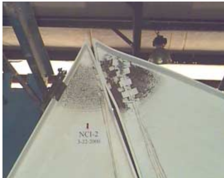
b) Yielding of Web on Tension Side
