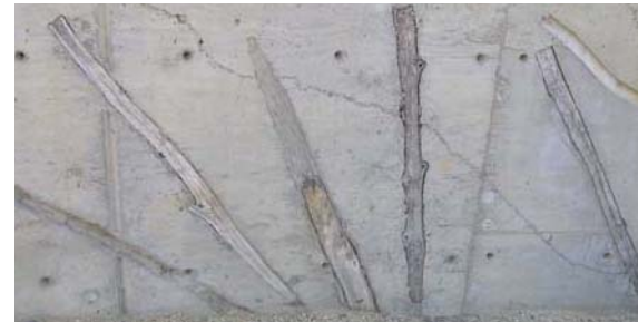
Wood forms embedded in the concrete wall around the rain garden.
