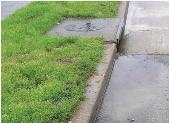
Water draining off the street into a sewer inlet after a storm.
