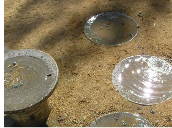
Splash pads collect water that drips off the pavillion roof.
