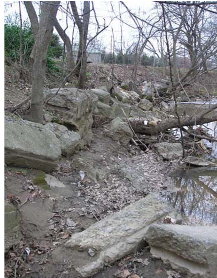
Typical view of eroding streambank.
