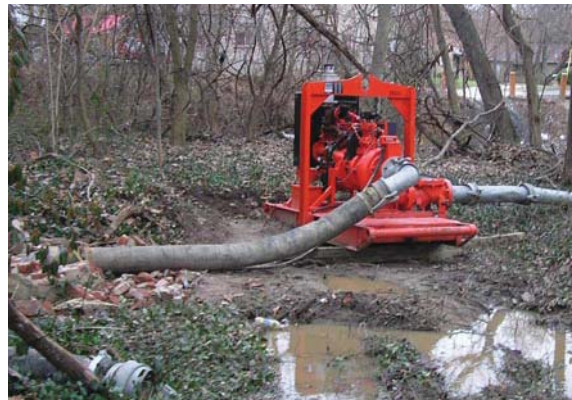
In addition to polluting the stream, the sewage spill on Martin Luther King Day 2006 resulted in damage to the riparian vegetation. Image shows pump intended to divert sewage from a broken sewer pipe.
