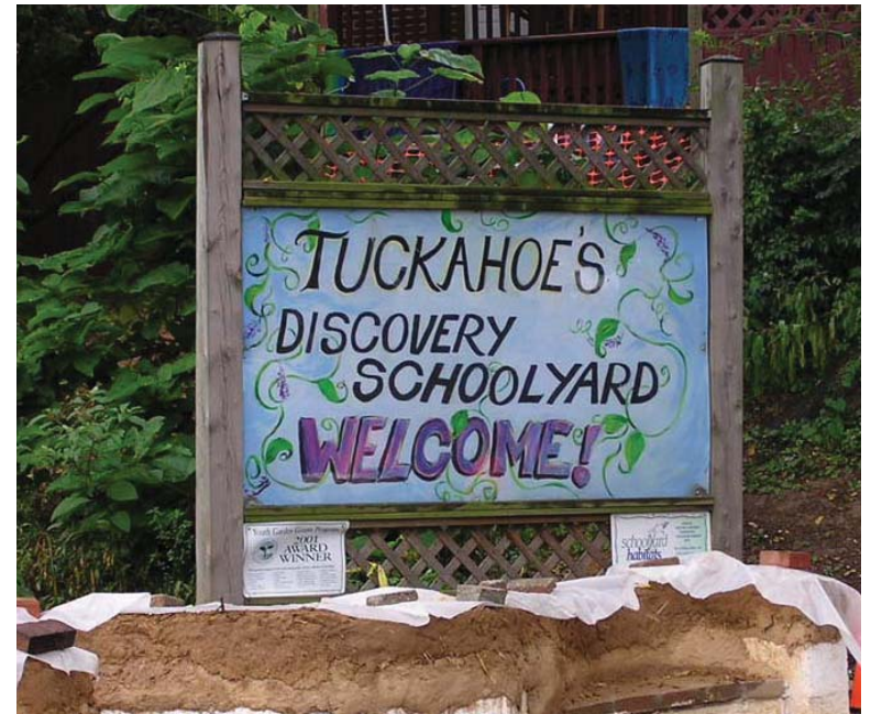
Welcome sign and cobb wall (in progress) made with the help of students.
