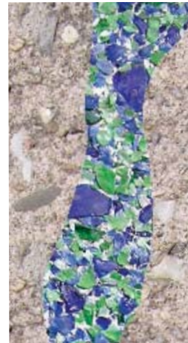
Detail of recycled glass inlay in concrete sidewalk.
