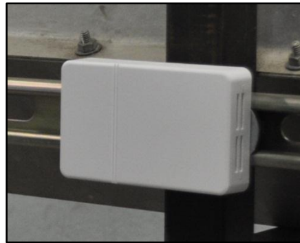
FIGURE 4.10. RELATIVE HUMIDITY/ TEMPERATURE SENSOR (WALL-MOUNT HOUSING)
