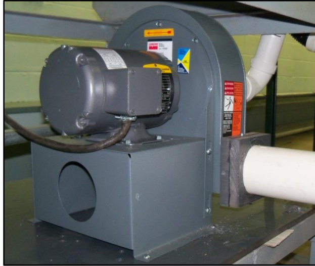
FIGURE 4.16. A 1/2-HP BLOWER FAN WAS SELECTED TO REPLACE THE SMALLER CENTRIFUGAL FAN
