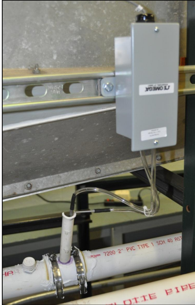
FIGURE 4.9. DIFFERENTIAL PRESSURE TRANSDUCER, CONNECTED TO PITOT-STATIC TUBE VIA TYGON PRESSURE TUBING
