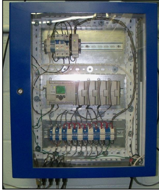
FIGURE 4.15. ELECTRICAL ENCLOSURE WITH ALL CONNECTIONS COMPLETED
