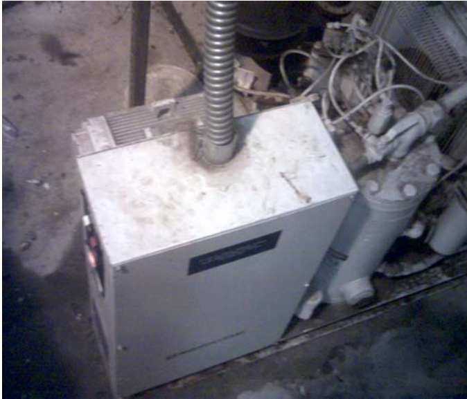
Fig. 1 Big air compressor
