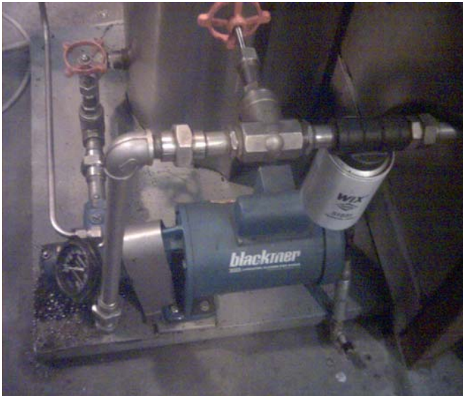
Fig. 8 Oil pump with isolation valves
