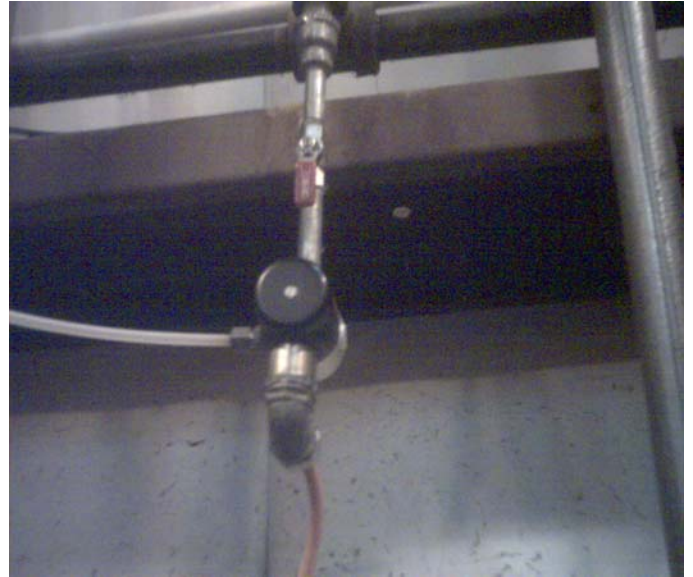
Fig. 2 Control air manual valve & transmitter
