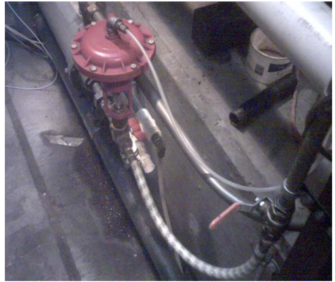
Fig. 5 Manual and Pneumatic valves
