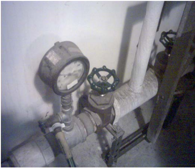
Fig. 4 Main valve with gauge
